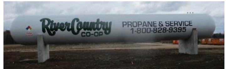
New propane plant in Hatley, WI.
