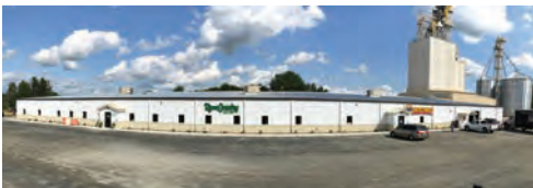
Owen Main Office & Feed Complex
