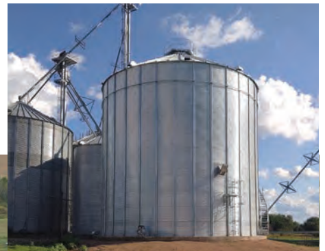
New 60,000 bushel bin constructed in Athens.
